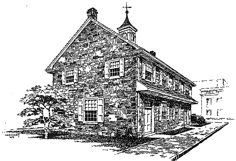
1724 Chester Court House, viewed from the southwest
