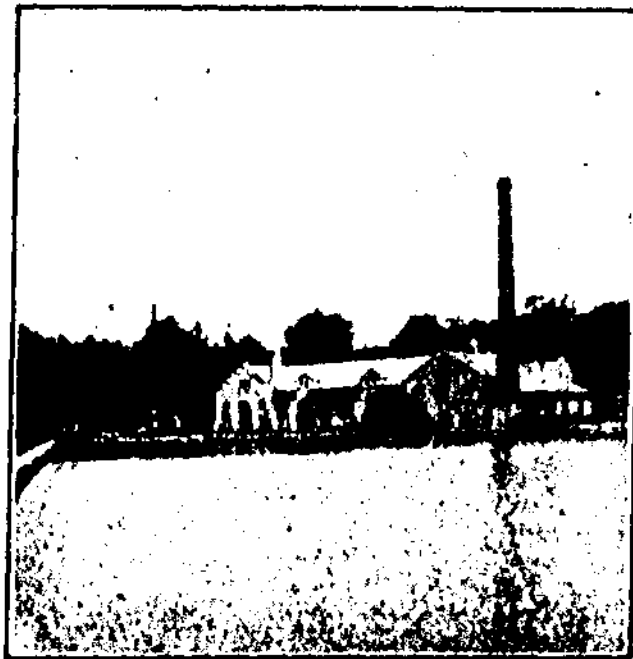
PUMPING STATION, SPRINGFIELD CON. WATER CO. MARPLE HILL, DELAWARE COUNTY.
